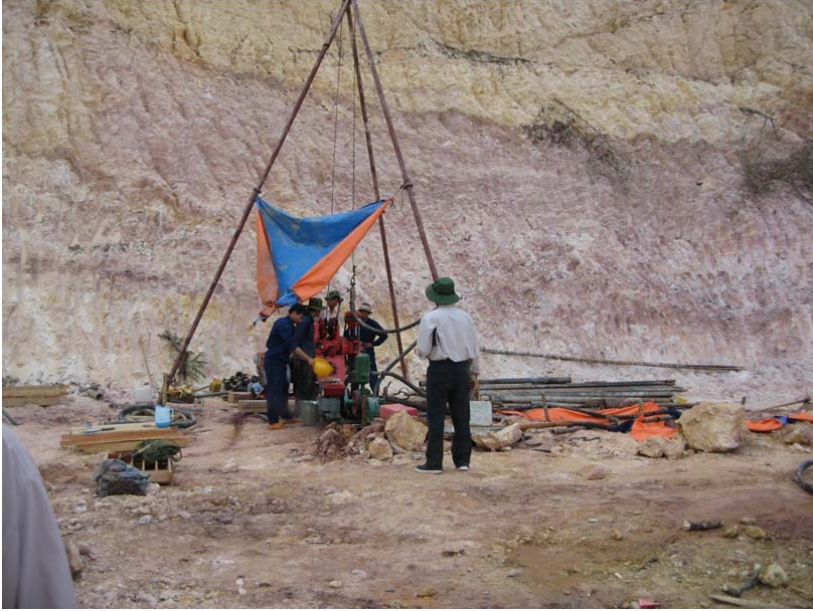
Picture II- 1:Drilling rig LK 2-T15
