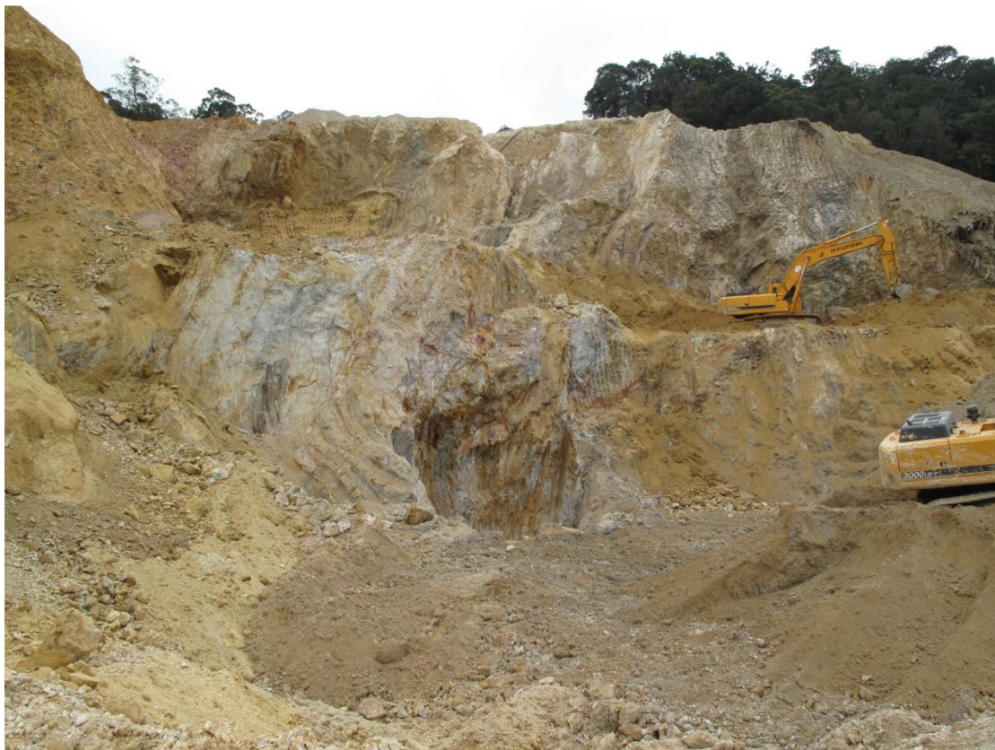
Photo III - 18: Trace Route A.0012 present northern part of the gold bearing dyke
